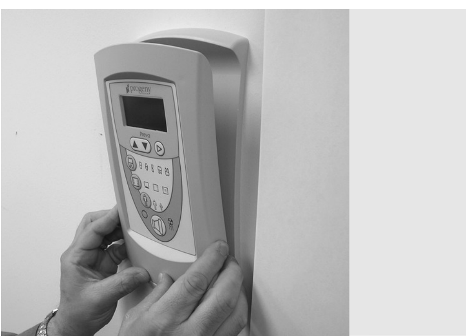
Figure 31 Snapping the Operator Panel to the Mounting Cradle
