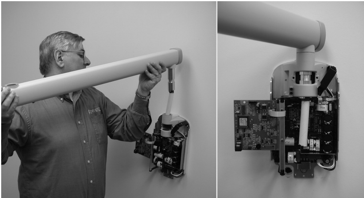
Figure 16 Installing the Horizontal Arm
